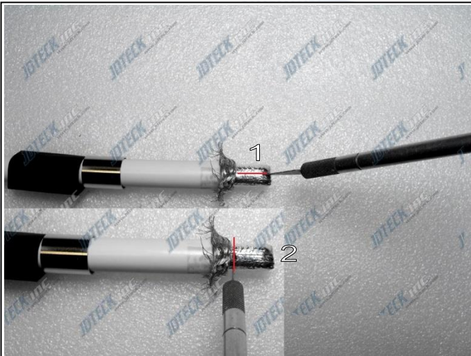
Use blade to score foil. (Laterally & Vertically)
